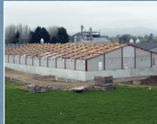
Piggery Building Complete
