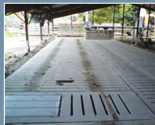
Replacing Old Slats
