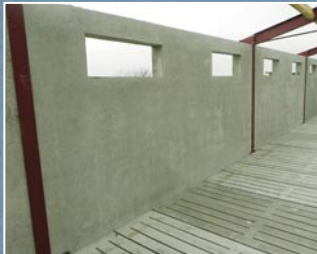
Insulated Pig Wall Installed
