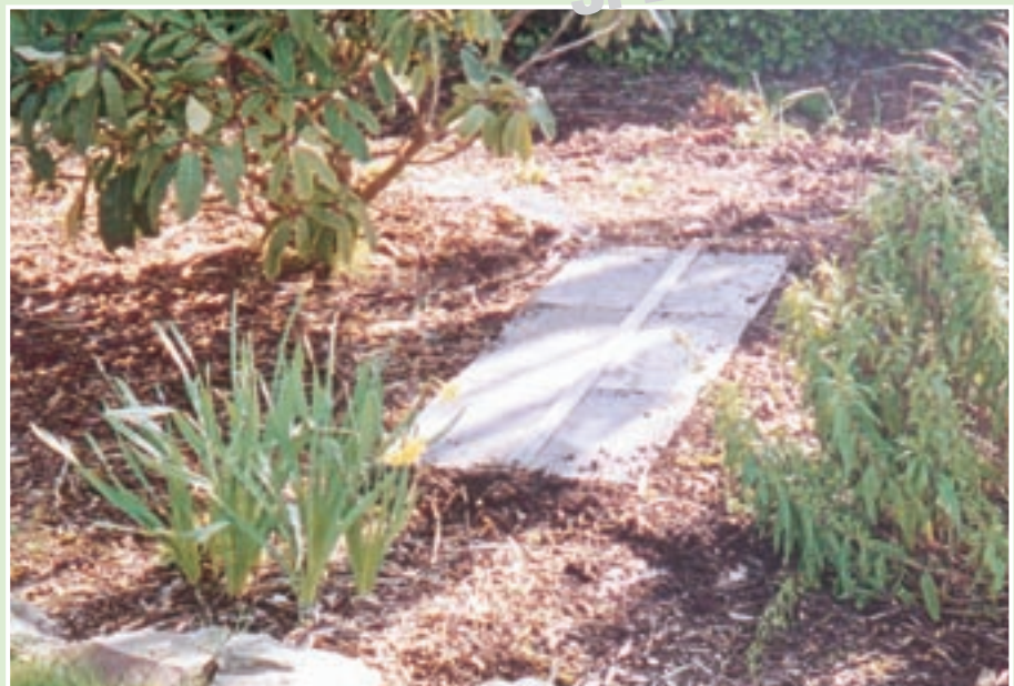
Photo showing tank cover
